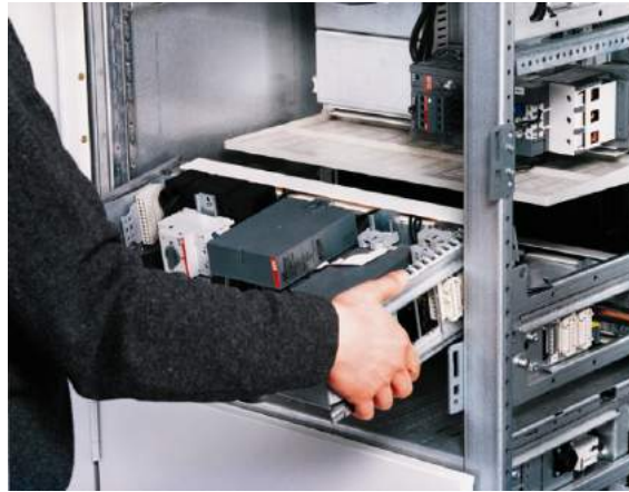
Fig. 62 Removal of a railable module:
